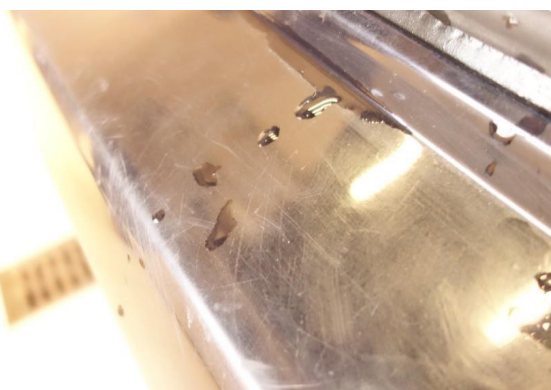
1.1 Riper innlasting baggagerom poleres
