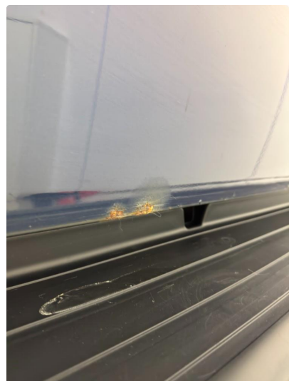
1.2 Diverse lakkskavanker / rust
