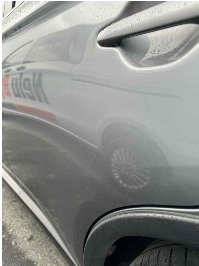
1.1 Noe riper i lakk
