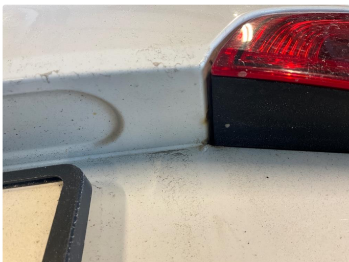
1.2 Rust i fals.
