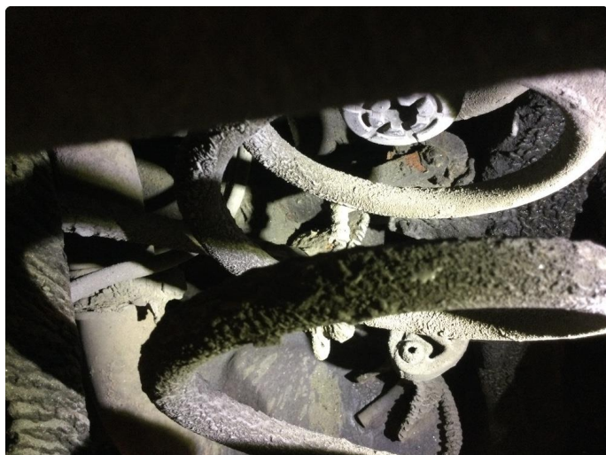
1.2 Noe rust, anbefaler behandling
