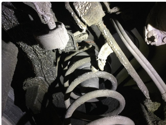
1.2 Noe rust, anbefaler behandling
