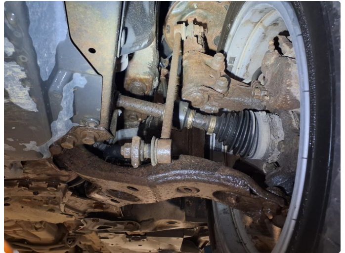
1.1 Overflaterust i understell
