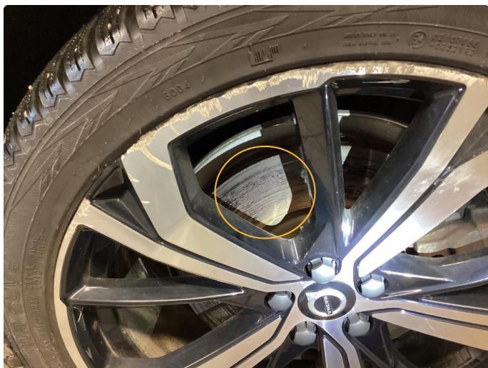
4.1 Mer enn 25% rust.OK
