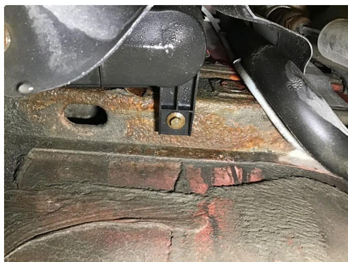
1.1 Rust underside bil.
