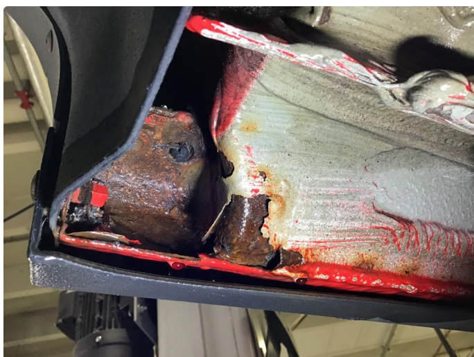
1.1 Rust underside bil.
