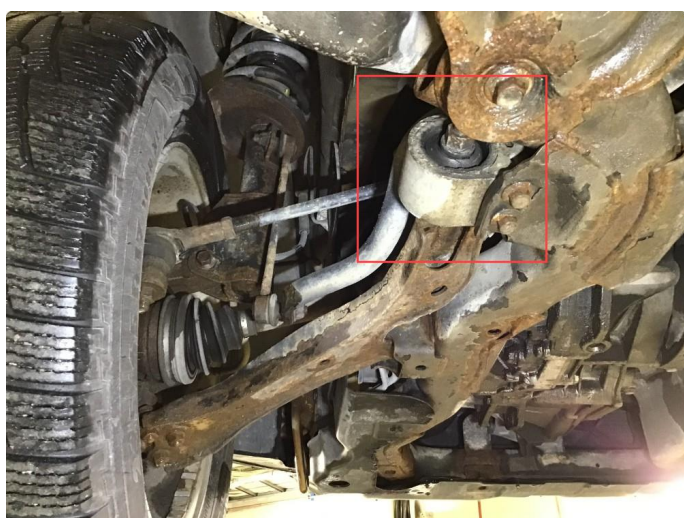
4.1 Utslitt casterforing h+v fram.
