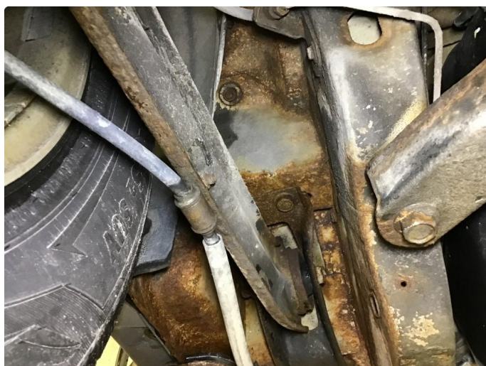
1.3 Mye rust underside bil.
