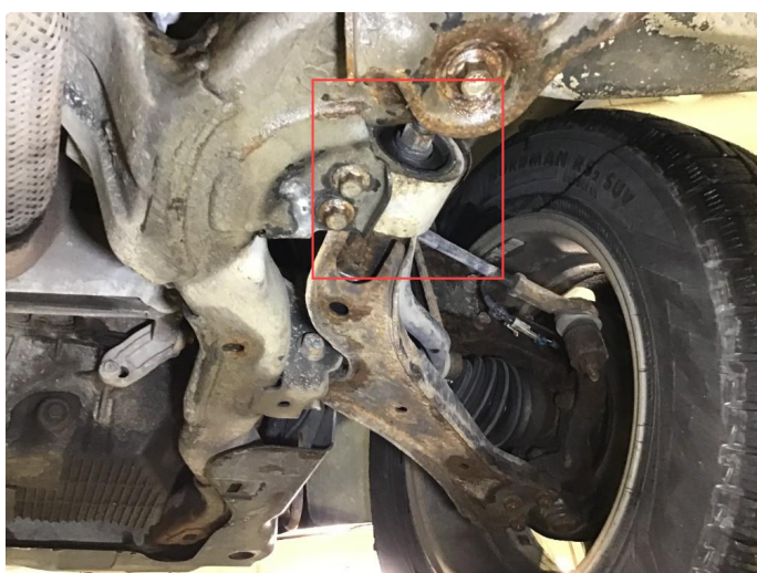
4.1 Utslitt casterforing h+v fram.
