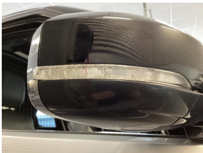
2.1 Krakelering i plast
