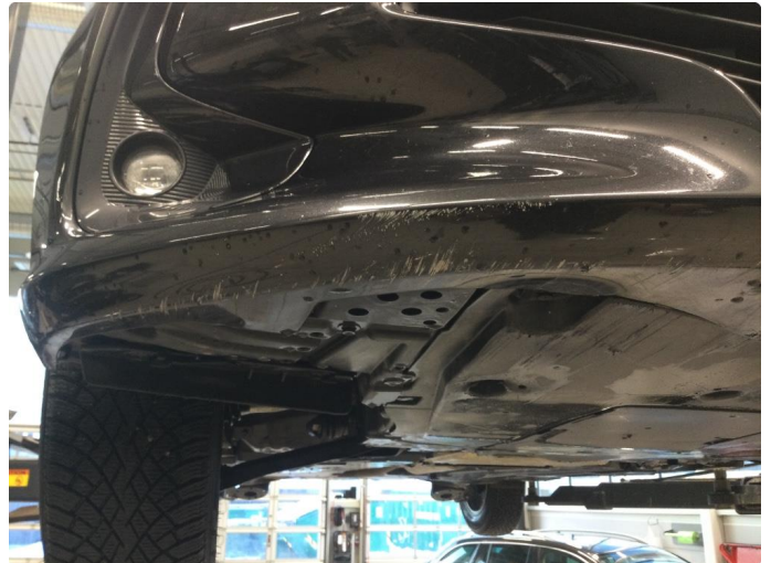
1.4 Skrubbskader underkant frontfanger
